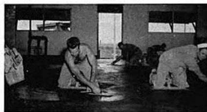
FINISHING CONCRETE
